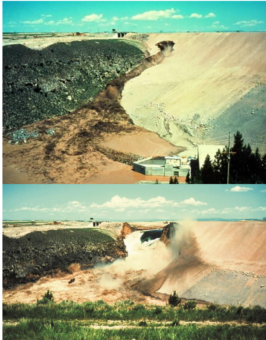
Fig. 2.13. Teton Dam failed on June 5, 1976. The failure released nearly 300,000 acre feet of water, then flooded farmland and towns downstream with the eventual loss of 14 lives and with a cost estimated to be nearly $1 billion. Photo by Mrs. Eunice Olson.
