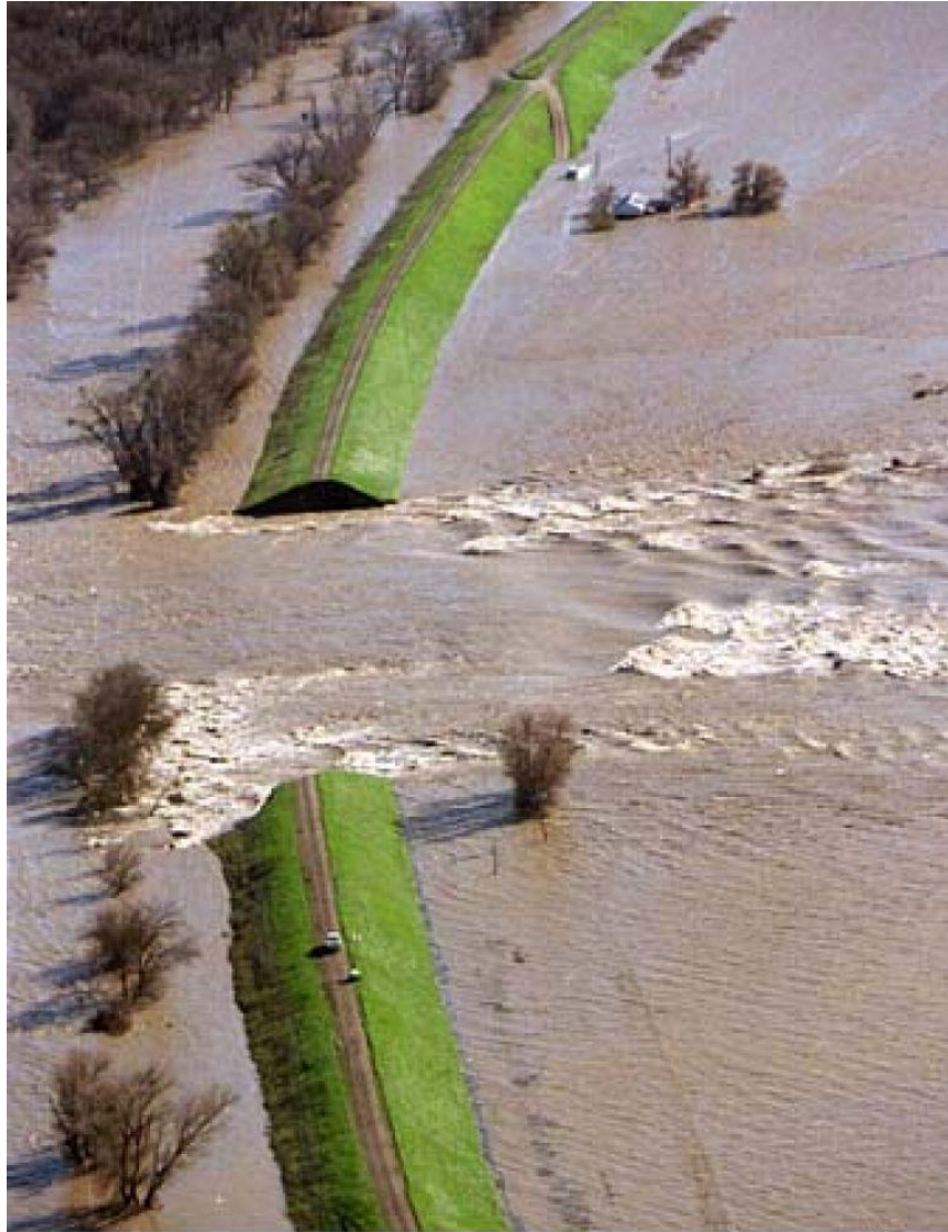
Fig. 7.25. Photo of Sutter Bypass Levee Breach ( http://ww3.hdnux.com/photos )
