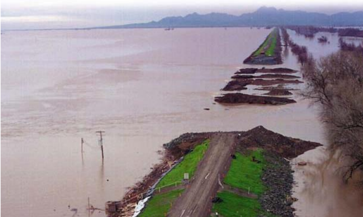
Fig. 7.26. Relief Cut of the Levee at the South End of the Meridian Basin Developed to a Full Breach (Photo taken three weeks after the breach)
